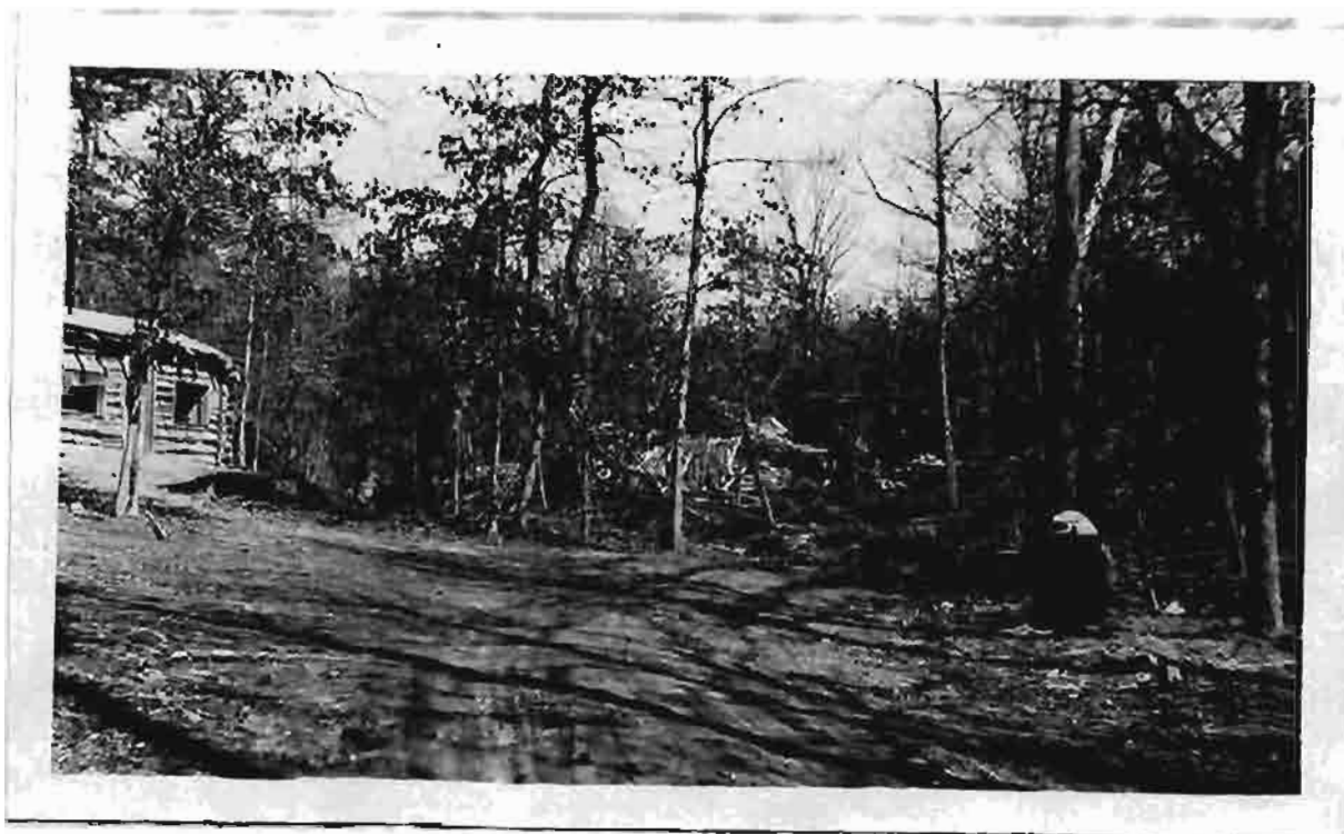
Figure 3. One of the many small sawmills in this area. Sec. 30, T.37 N., R.1 W.
